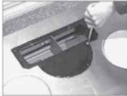
2. Place rectangular transition adaptor as shown by first installing 4 screws on half round section.
