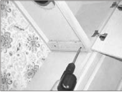
5. Reinforce cabinet base with 1x2 wood strips if additional strengthening is required. Unscrew and remove bottom grease splash shield.
