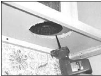
4. Cut out cabinet base opening if necessary.
