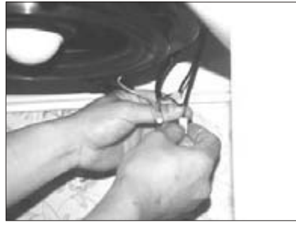
12. Connect both wires (blk) on hood to either power supply (blk or wht). Ground green wire.**
