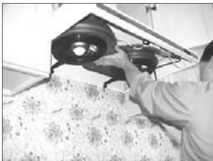
9. Fasten front of hood. Level all sides and adjust accordingly.**
