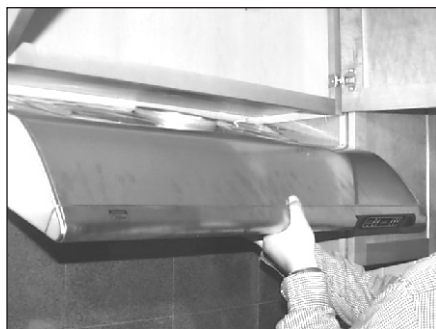
11. Lift hood and hook rear opening slots onto 2 rear brackets previously installed on wall
