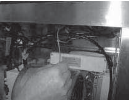
9. Use plastic tie to hold wiring together.
