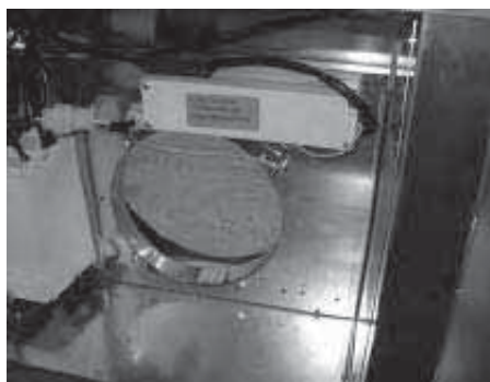
9. Attach grounding wire from external blower wiring box to grounding screw of the junction box. Refer on Fig-A in diagram below.
