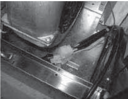
7. Attach short capacitor connector to blower connector.
