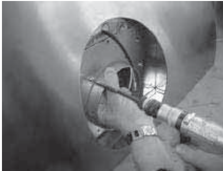
2. Attach blower to flange as shown using the provided 1/2" 5x15mm screws with washers.
