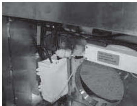
8. Attach connector from external blower wiring box to control board box connector inside hood.
