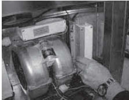
3. Position capacitor box as shown.
