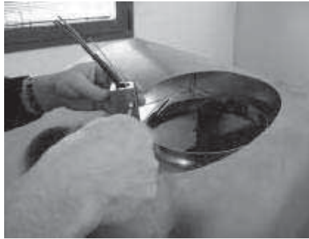
7. Secure cover to box with provided screw.
