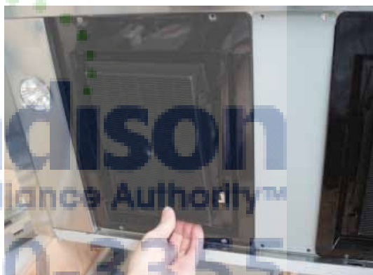
3. Install charcoal filters into charcoal filter brackets
