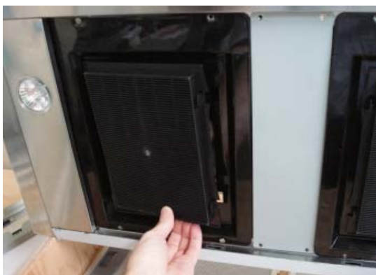
4. Install charcoal filters into charcoal filter brackets
