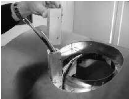
6. Position cover onto external blower wiring box.
