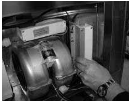
3. Position capacitor box as shown.
