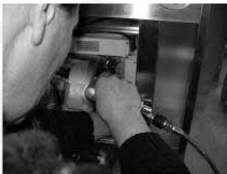
4. Secure capacitor box to hood using the provided 1/2" self tapping screws.
