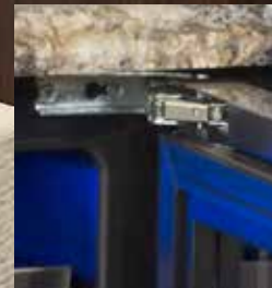
Soft-Close Integrated Hinge
