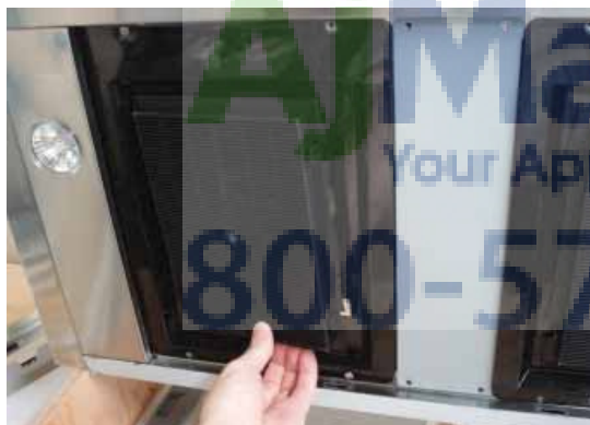
3. Install charcoal filters into charcoal filter brackets
