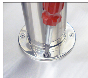
FIG. 3. Secure the draft standard to the countertop.
