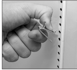
FIG. 1. Installing top tab of shelf clip.
