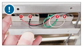
FIG. 5. Label the original wire locations **BEFORE** disconnecting the reed switch.
