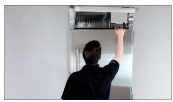
FIG. 3. Be sure to inspect behind the rainshield.
