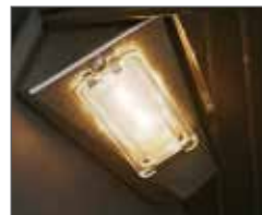
Interior Lights for Late Night Entertaining
