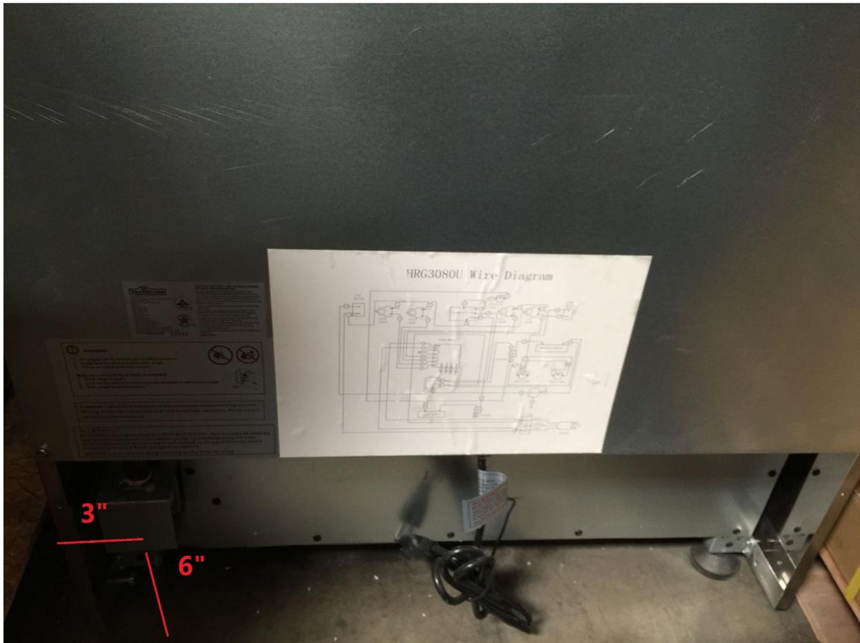
Distance from inlet gas pipe to right side of the range is 3".
