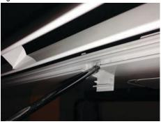
Figure 57: Indoor Unit Knockout (Communication Wires)
