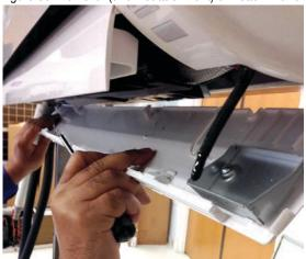
Figure 54: Latch over Screws on Bottom Panel, Indoor Unit
