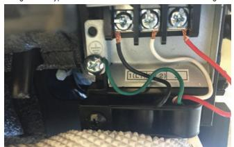
Figure 59: Typical Indoor Unit Terminal Block Connections
