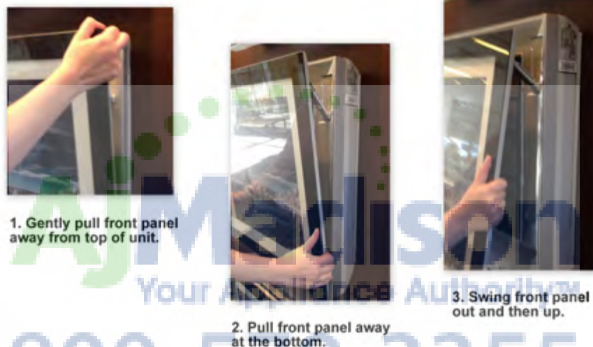
Figure 12: Lifting of Front Panel from Indoor Unit
