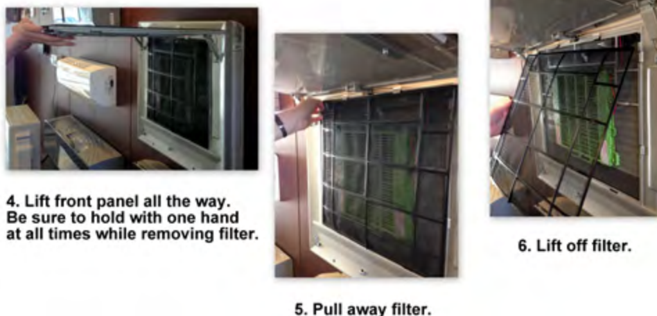
Figure 13: Detaching Filter from Indoor Unit
