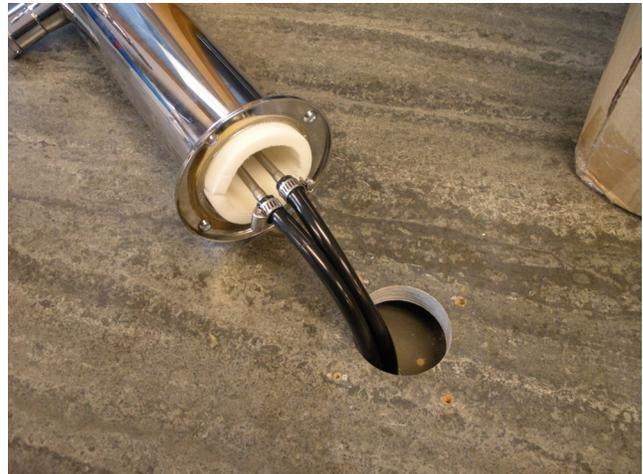
3. Using the 3/8" -thick foam pad included in the tapping kit and roll into a cylinder. From inside the cabinet, insert the foam tube up through the hole in the counter top until it is firmly against the insulation in the dispensing head. Cut away any excess foam that extends into the cabinet that extends into the refrigerator.
