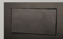
CONCEALED CONTROL PANEL
