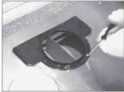
1. Remove pre-mounted 7" transition adaptor or duct opening.
