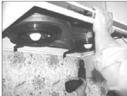
8. Support hood to place, fasten both rear with screws and washer provided.
