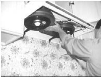
9. Fasten front of hood. Level all sides and adjust accordingly.**
