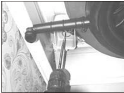
10. Drill out cabinet base through electrical box with 3/4" boring bit.
