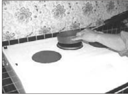
6. Install damper if required by local codes (not provided), or install 6" starting collar (green).**
