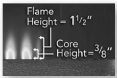
Flames should be blue and stable with slight yellow tips. The bright-blue core should be about 3/8 inch high with a total flame height of about 1 1/2 inches.
